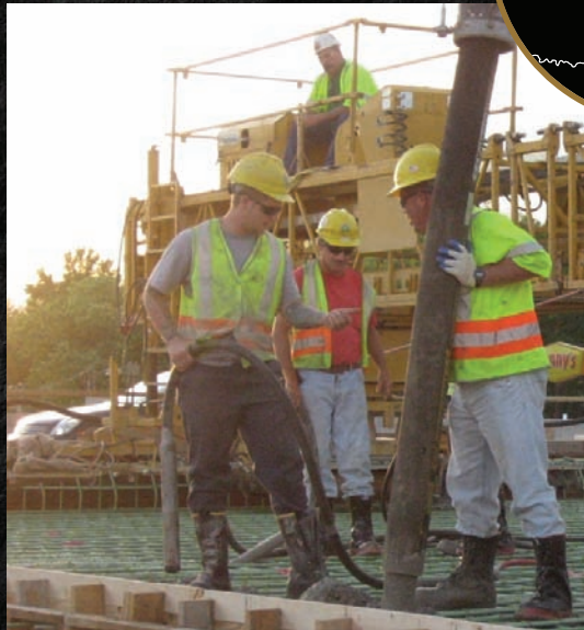
PHOTOS COURTESY THE MISSOURI DEPARTMENT OF TRANSPORTATION.
